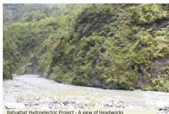
Rahughat Hydroelectric Project - A view of Headworks
